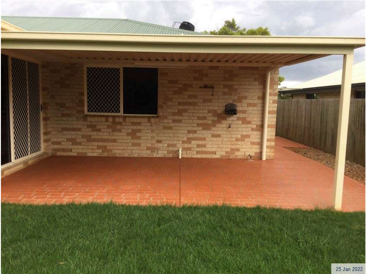
Outdoor Covered Area
